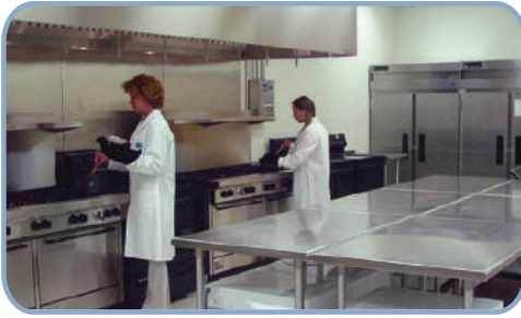
commercial test kitchen
